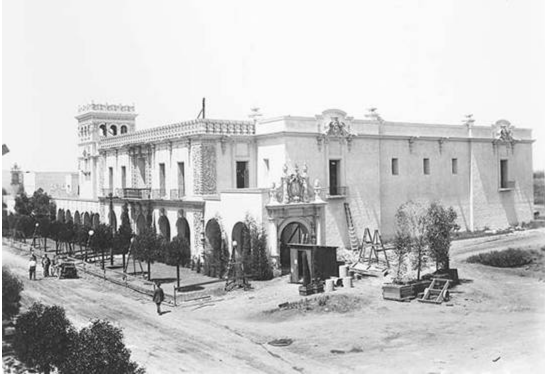
Home Economy Building, East Side under Construction
